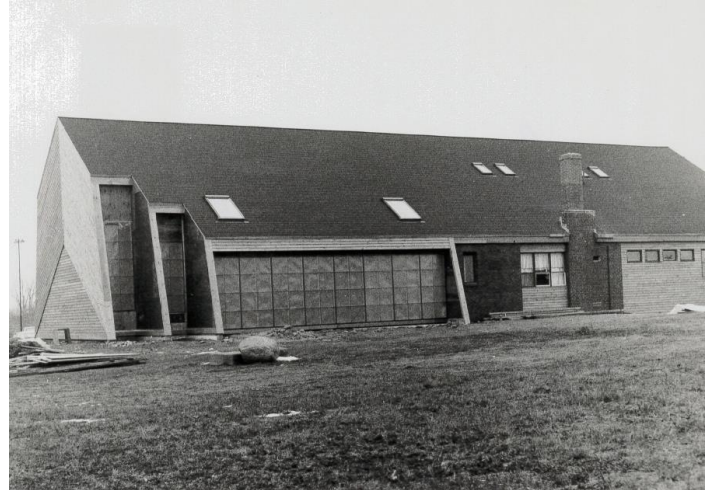
Passive Solar Wall Facing South
